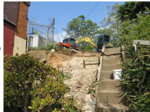
Above: The old fire escape removed with foundation preparation under way.
